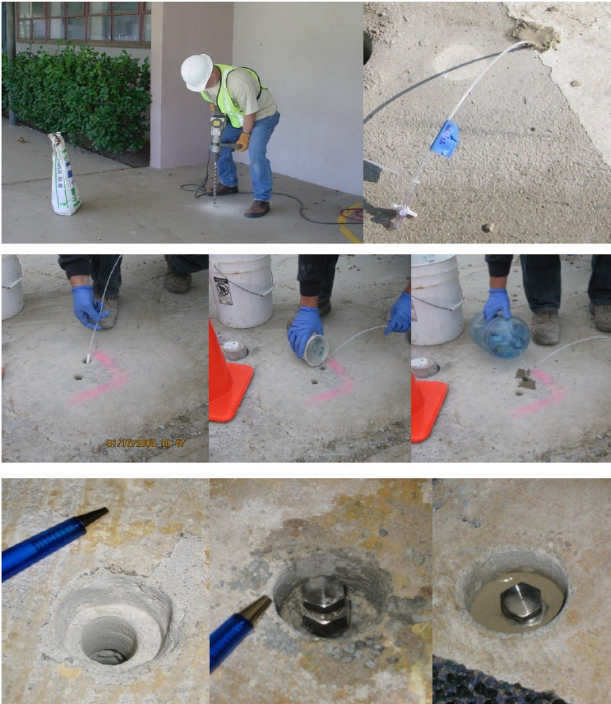
Figure 7 Figures showing installation of permanent sub-slab sampling probe.
